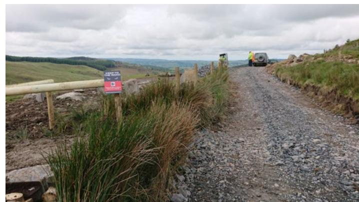
In total, 1,000 tonnes of material was used to repair a 1.75km length of the track, creating a level surface without ruts or holes. Infill material was used to reinstate the surrounding land, and stone was added to the surface. Drainage channels and ditches were dug to allow surface water to run off the route in order to maintain the surface during adverse weather. Pipes were re-opened, connecting to nearby drainage ditches so that water can be removed from the area.
